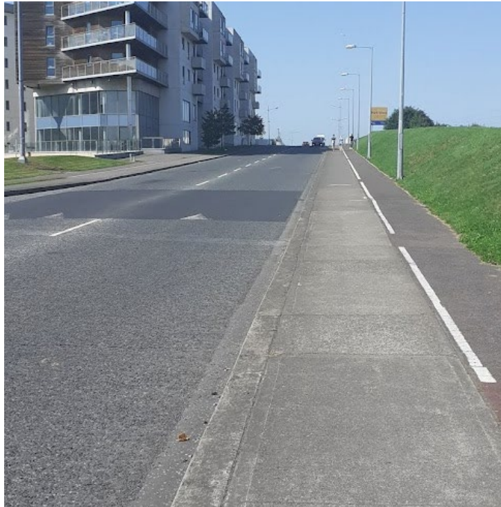
Figure 14- Crest in road for railway bridge
