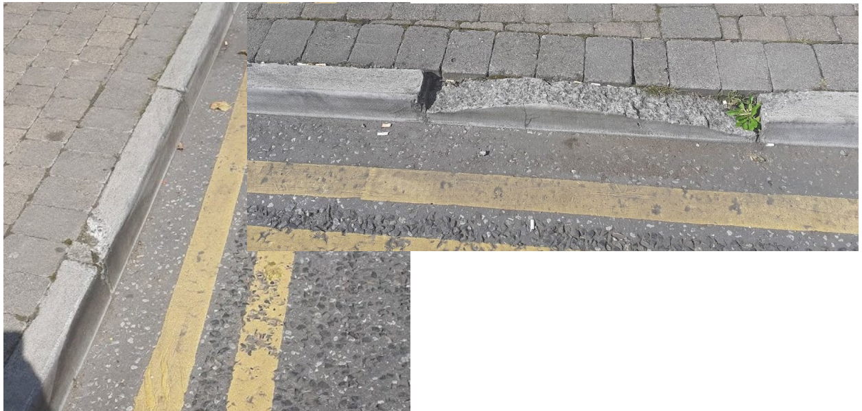
Figures 9-10 – Kerbs Damaged by HGVs
