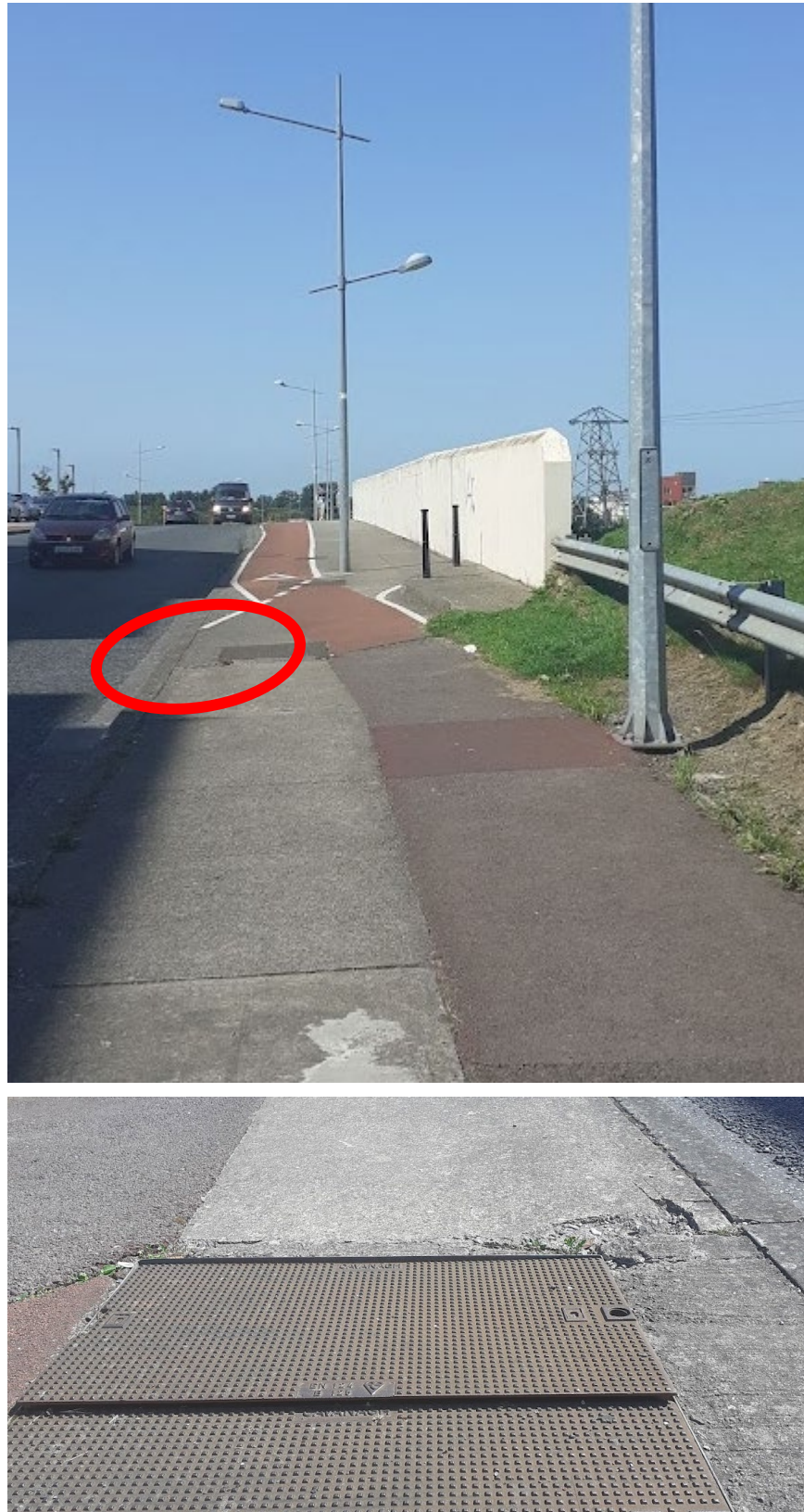
Figure 17/18 – Damaged Chamber lid
