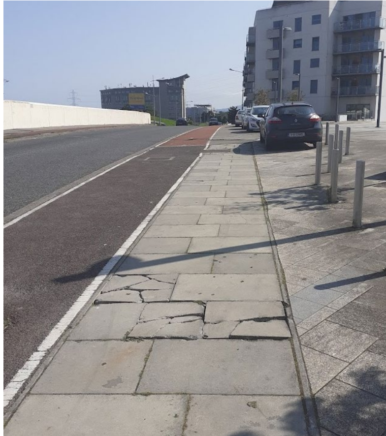
Figure 19 – Damaged paving caused by informal parking
